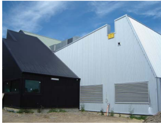
fig. 123: Knox Leisureworks Pool addition, East annexes during construction, 2010
