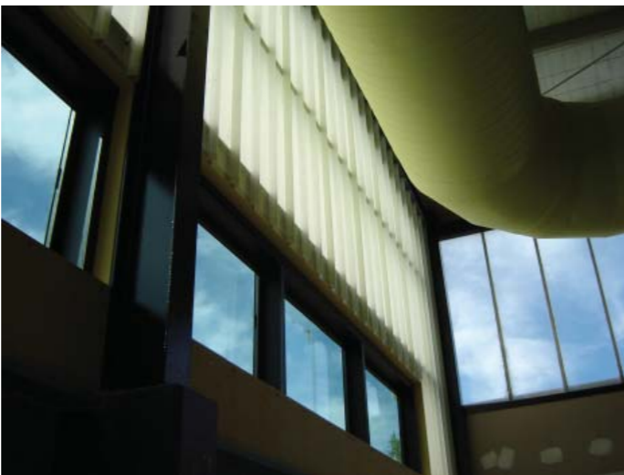
fig. 124: Knox Leisureworks Pool addition, during construction, 2010
