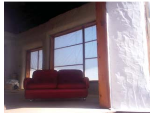
fig.148,149 : Strawbale House, informal inhabitation during construction.
