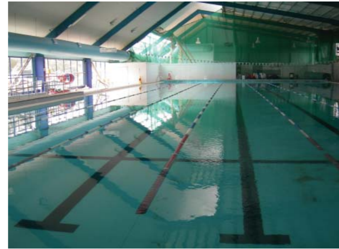
fig. 122: Knox Leisureworks Pool addition, 50m pool during construction, 2010
