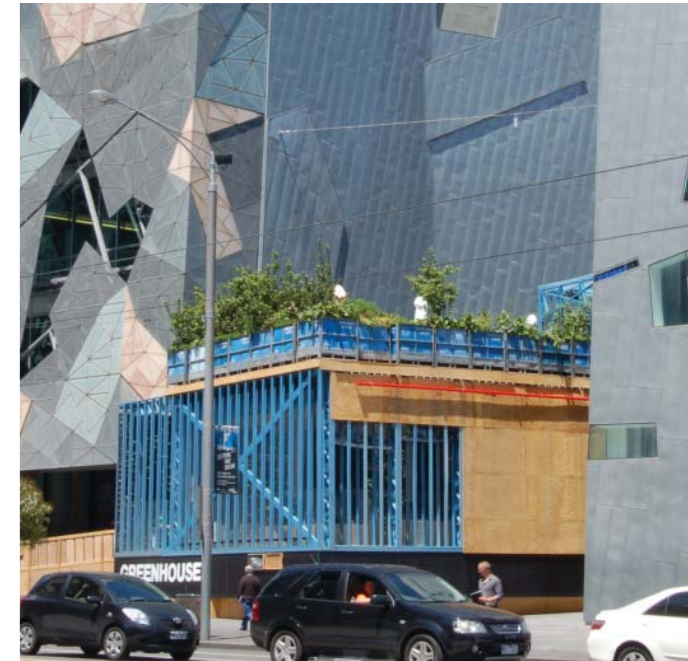
fig.140: Greenhouse at Federation Square, seen between the zinc clad buildings
