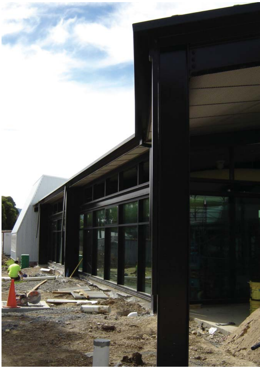
fig. 120: Knox Leisureworks Pool addition, during construction, 2010
