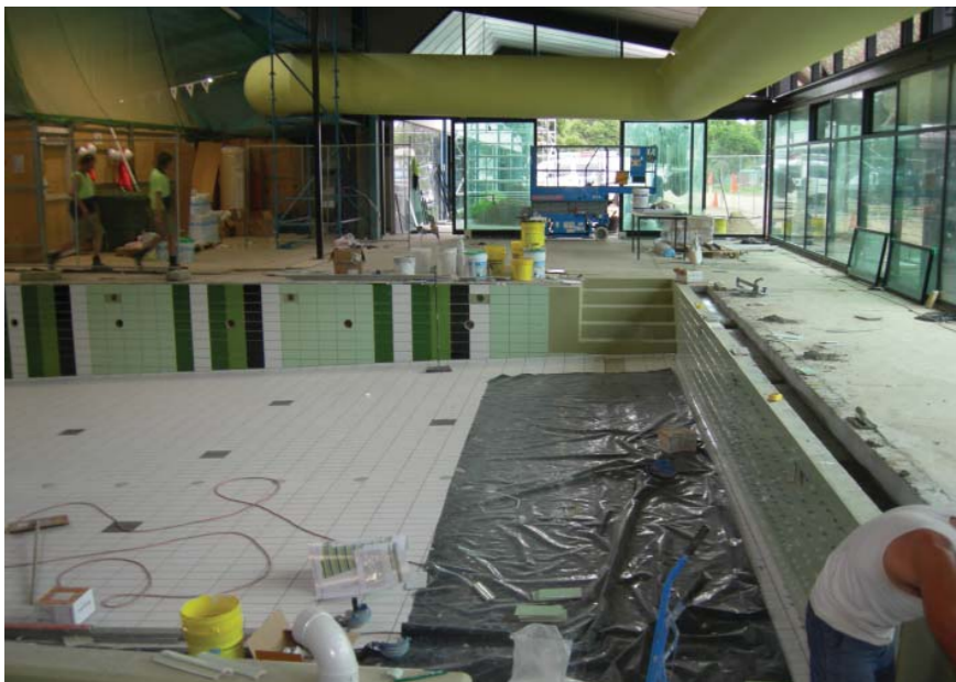
fig. 121: Knox Leisureworks Pool addition, during construction, 2010
