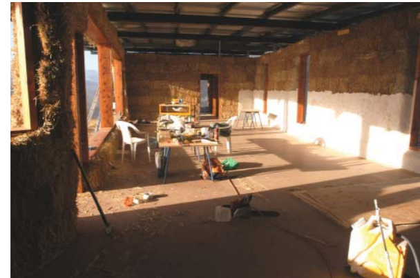
fig.147 : Strawbale House, interior during construction.
