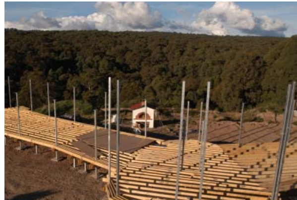
fig.146 : Strawbale House, framing construction.
