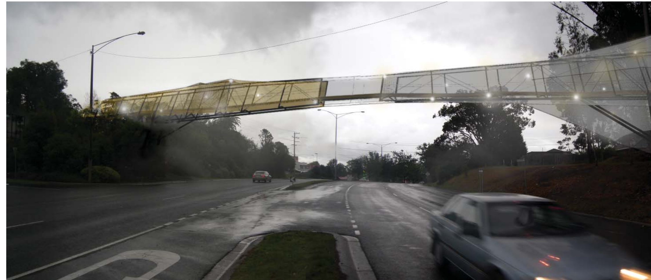
fig. 113: Warburton Trail Bridge; view from the highway.
