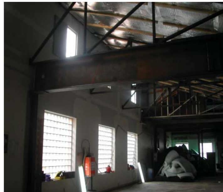
fig.137: The Reach Foundation, interior of the theatre space during construction.
