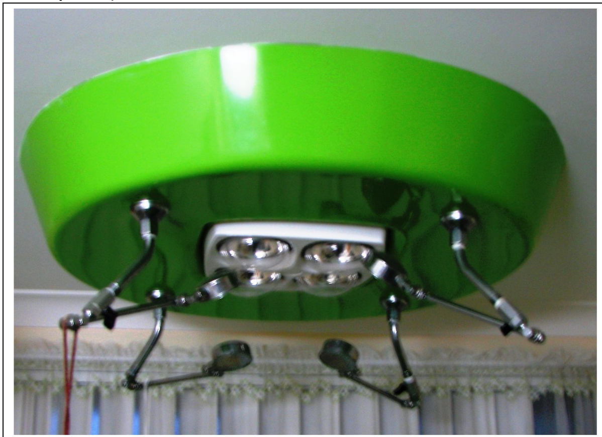
Figure 1.3: A non-efficient quadruple showerhead array with four heat lamps (flowing over a spa bath)
