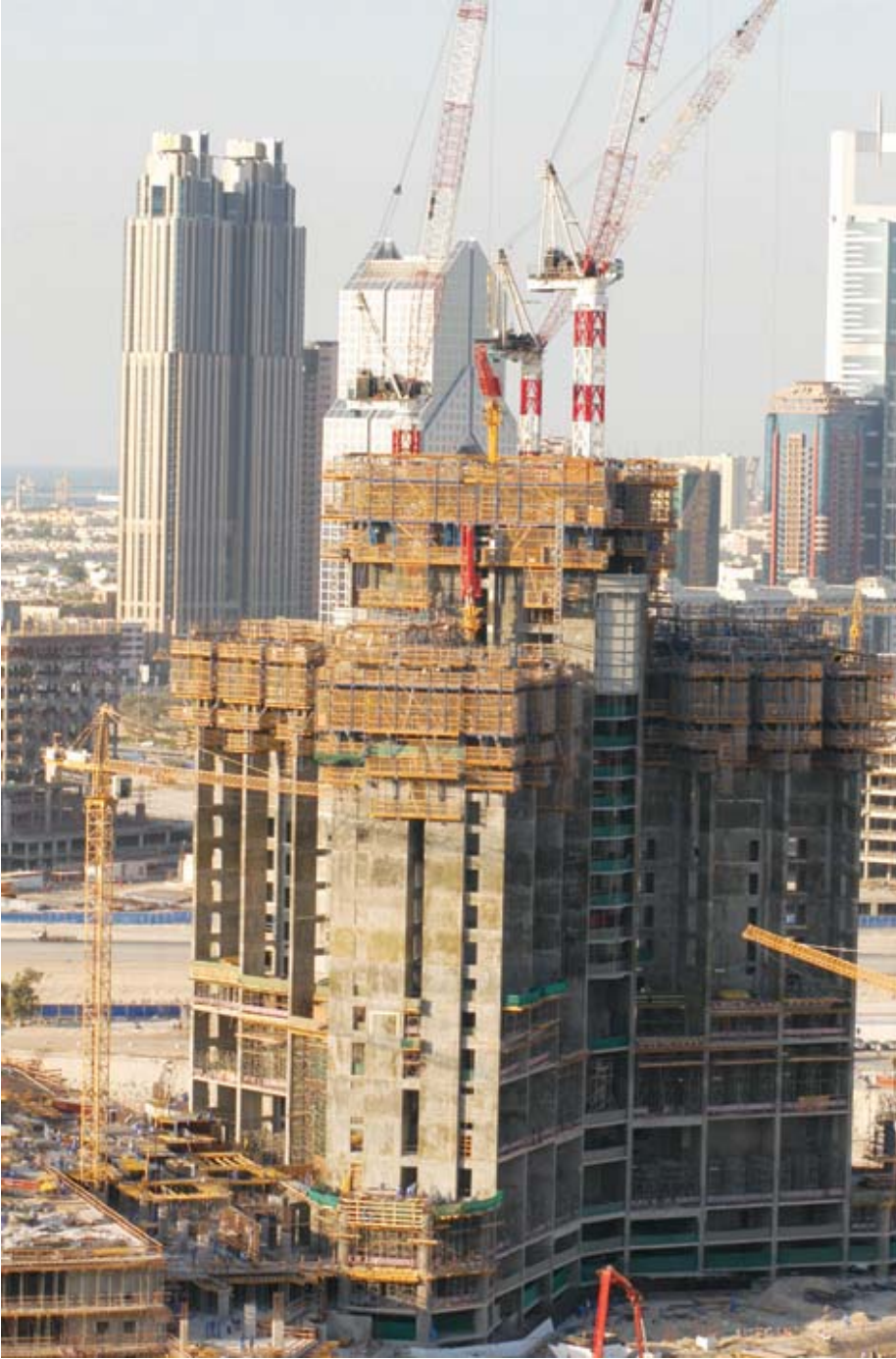
Figure 2. Dubai Tower under construction (Image courtesy of Bernadette Redfern)
