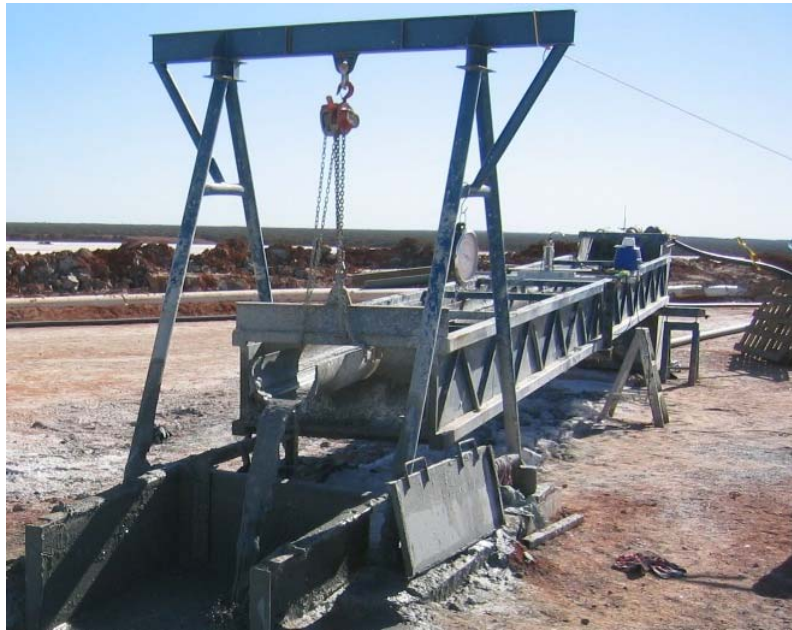
Figure 13. Trestle at downstream end of flume with chain block for raising/lowering of flume
