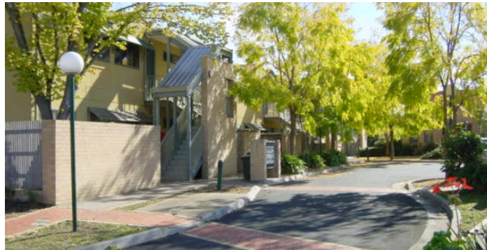
Figure 25: Image of public housing estate renewed under the ‘Better Cities’ program
