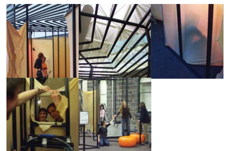
8.13 Constructing the installation structure.
