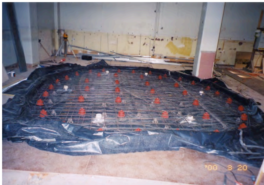
Image 47: The Pod during construction
