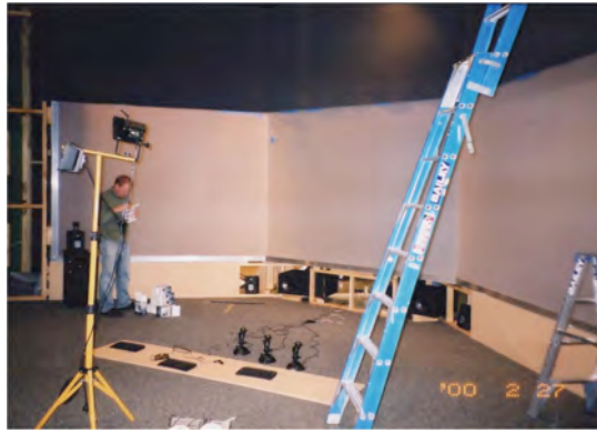
Image 11: Ecstasis Perth exhibition space during construction
