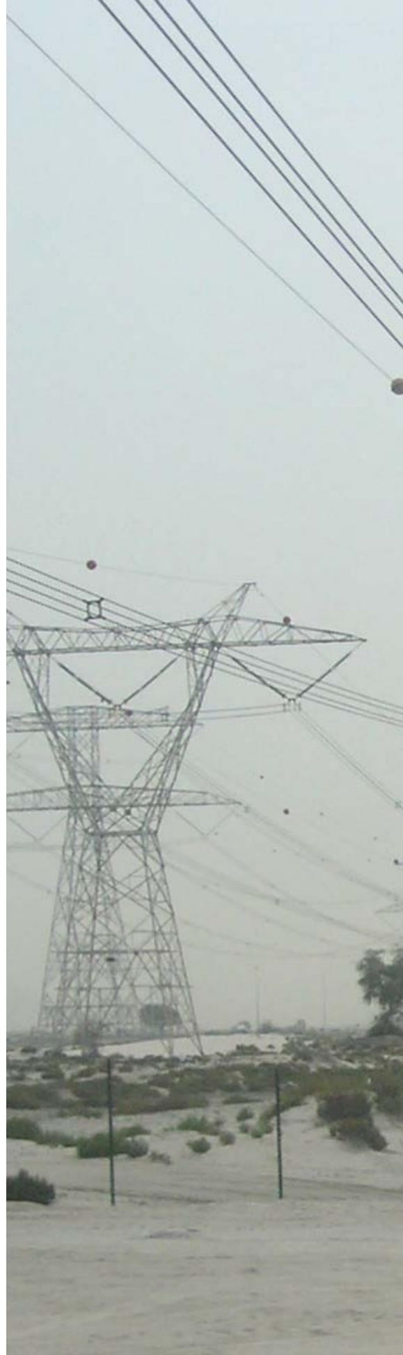
Powerlines, Dubai, United Arab Emirates.
