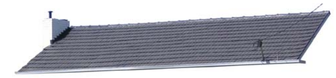
Impervious, angled roof for catchment of rain water
