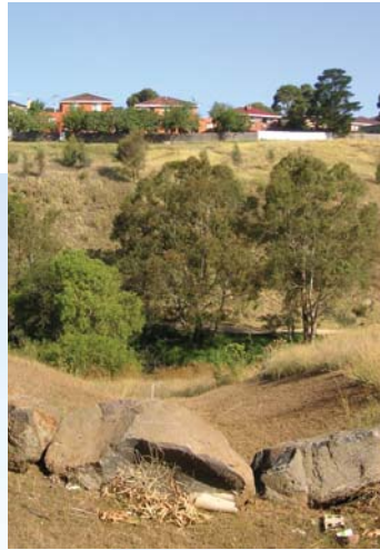
Rocks act as an inadequate gross pollutant trap for the swale before discharge.
