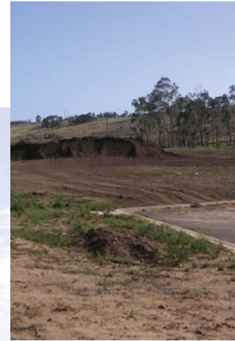
Soil stockpiles should be at least 10m from the river and have a surrounding silt fence or drainage system.
