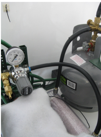
Figure 5-13. The air regulator and release valve set-up, as part of 500 W fuel cell air supply line (see figure 5-10)
