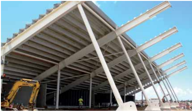
Steel structure and concrete slabs on site
