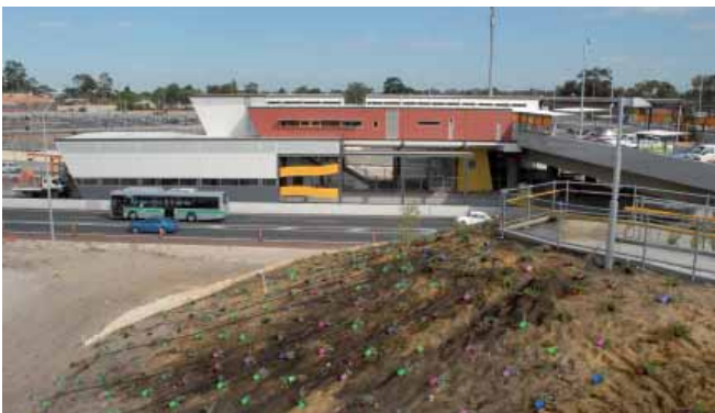
Completed Bull Creek Station (Source: New Metrorail 2006)
