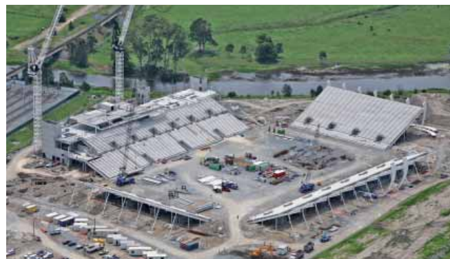
Robina Stadium site January 2007 (Source: Watpac Construction)
