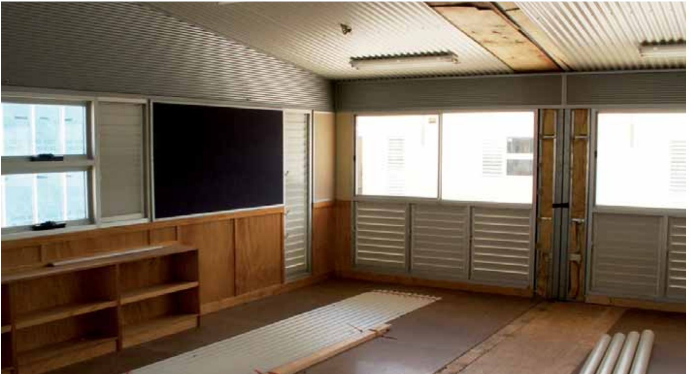
Completed classroom at factory showing cladding left off at module joints
