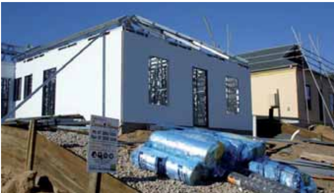
Construction on site (Source: Monarch)
