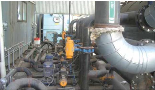
Boiler system used to accelerate curing of the moulded concrete
