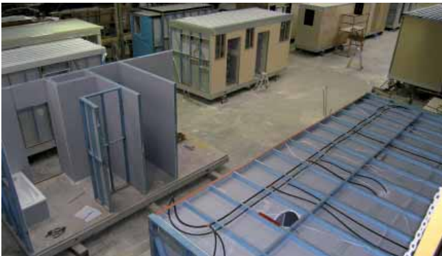
Bathroom modules in production (Source: Monarch)
