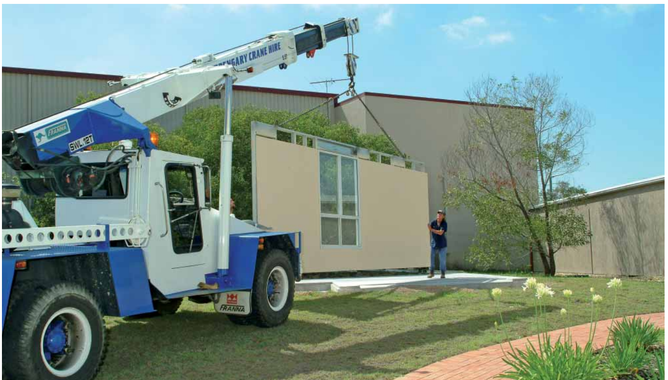
Lifting completed wall panels onto site (Source: Monarch)
