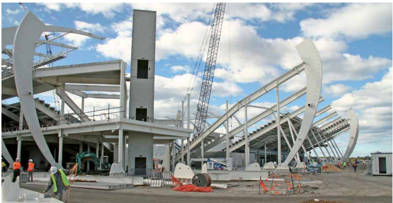
Off-site manufactured steel structures in place
