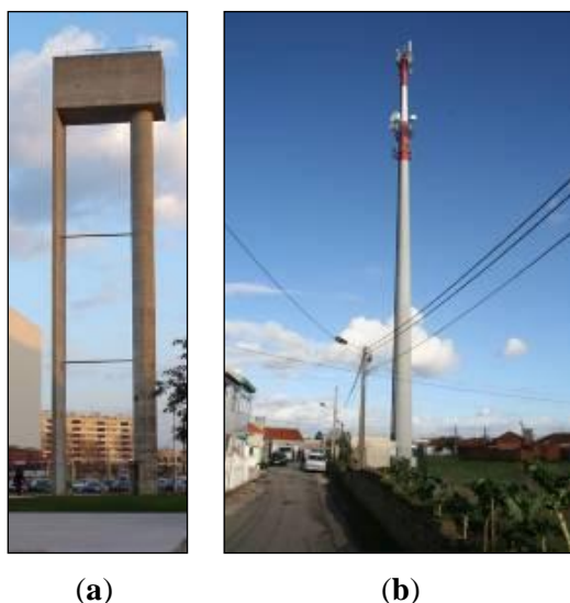
Figure 4. Photographs of the University of Aveiro water reservoir (a) and telecommunication tower (b).
