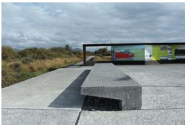
2016 The Marconi Station – Denis Byrne Architects The provision of visitor and interpretative facilities at the historic Marconi Telegraphy Station and Alcock & Brown transatlantic landing site on a bog near Derrigimlagh, County Galway.
