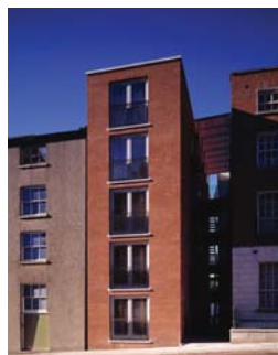
2004 Cigar Box – Denis Byrne Architects A mixed development of apartments and offices, beside the above building, where the main character has his offices and gallery. The front doors are 9 ms apart.
