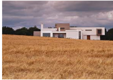
2008 House in a Field, Mullingar Denis Byrne Architects
