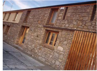
2002 Mews House, Dublin Denis Byrne Architects
