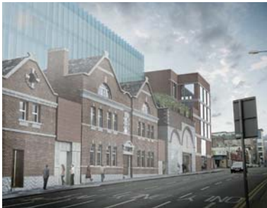
2017 Gardens International, Limerick Denis Byrne Architects with Carr Cotter Naessens Architects
