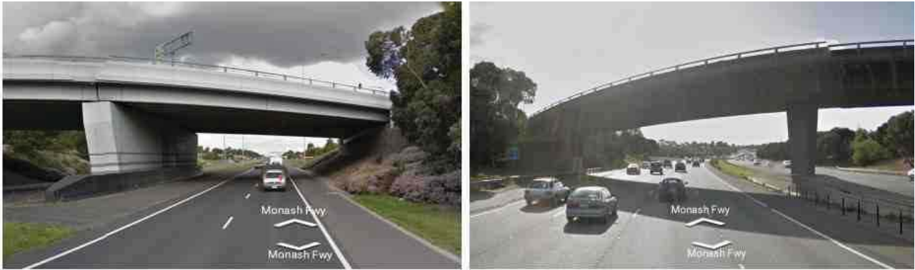
Figure 7-6: Examples of the environments where selected speed outliers were generated by Novatel GPS receiver with a 5° mask angle on Monash Fwy
