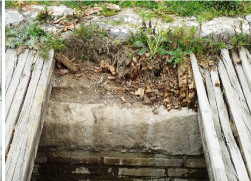
Fig. 4 - Bearing on stone elements ("B")
