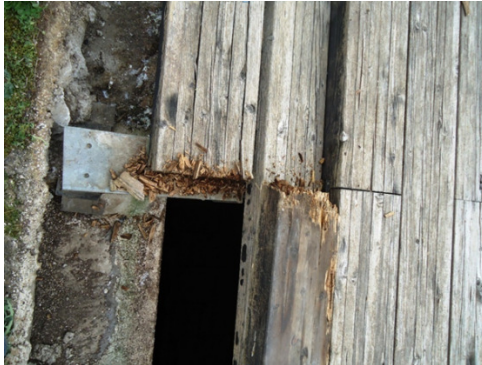
Fig. 3 - Bearing on steel profiles ("A")
