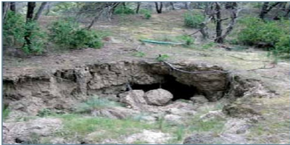
Figure 1.5 Piping failure of a dam. (Hardie 2009)
