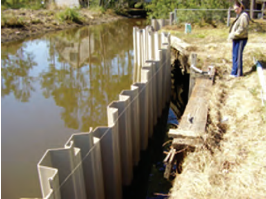
Figure 3.2. Example of vinyl bulkheads (adapted from Ecobuilders, 2012).
