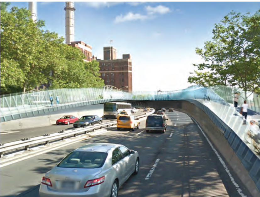
Figure 3.6. A proposed pedestrian and bicycle bridge at 14th Street forms a security and flood barrier for a substation while connecting to the waterfront (source: WXY architects).
