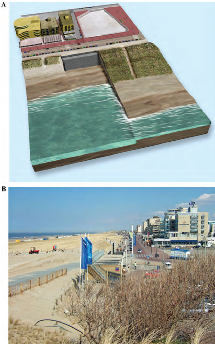
Figure 3.7. Model of a dike within a dune and beach strengthening project in the beach resort Noordwijk in the Netherlands ( Top ) (Adapted from: http://www.kustvisie.nl/noordwijk.php ). Photo of the dike within dune project in Noordwijk, just after completion ( Bottom ) (adapted from: http://www.hooijmans-noordwijk.nl/keuze/dijkaanzee.html ).
