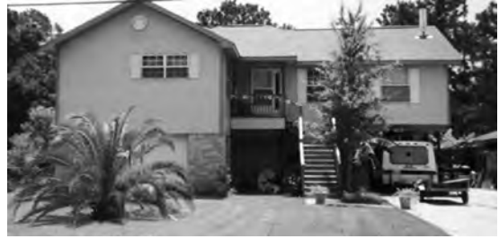
Figure 2.1. A house that is elevated using a continuous wall foundation (Source: FEMA, 2009b).
