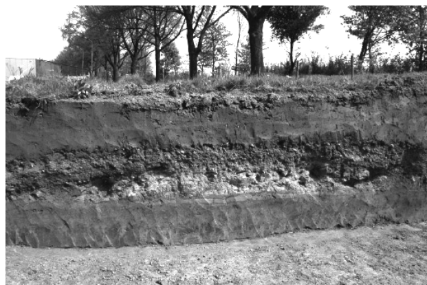
Figure 3 Cross section of the Via Belgica in the vicinity of Voerendaal.
