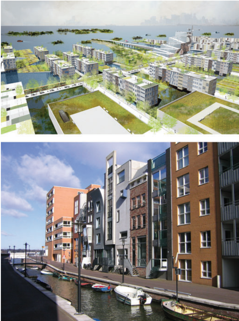
Figure 5.6. Artist's impression of southwest Brooklyn with Amsterdam style residential areas ( top ). Source: NArchitects (2010). Amsterdam, Java Island: a revitalized old port facility now converted into a residential area (Amsterdam, the Netherlands) ( bottom ).
