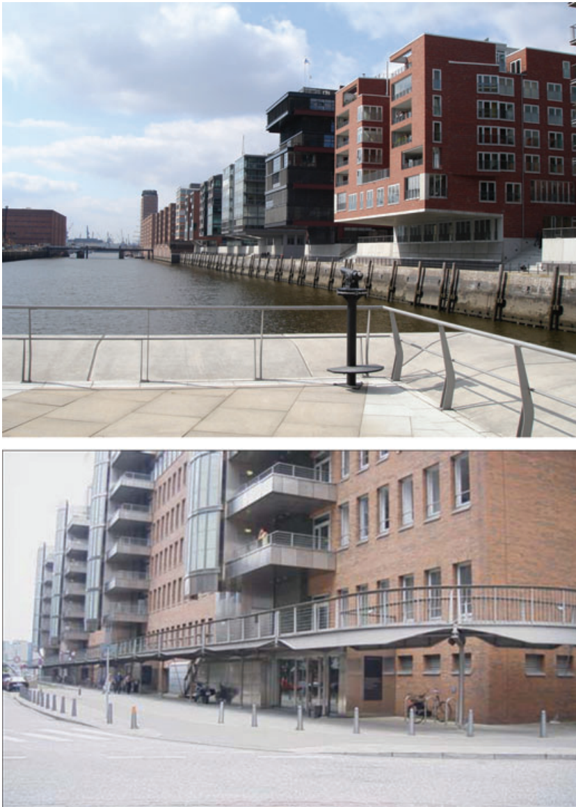
Figure 7.2. HafenCity (City of Hamburg, Germany) with the boardwalk at about 9 ft and the residential apartments at a level of 22 ft (top). Emergency serviceway above the design water level at HafenCity (bottom). Source: Jeroen Aerts.
