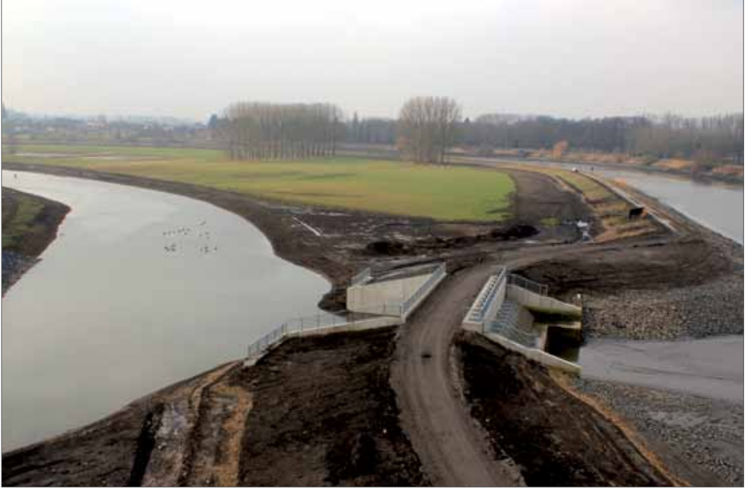
Figure 4.3. CRT sluice and stream source
