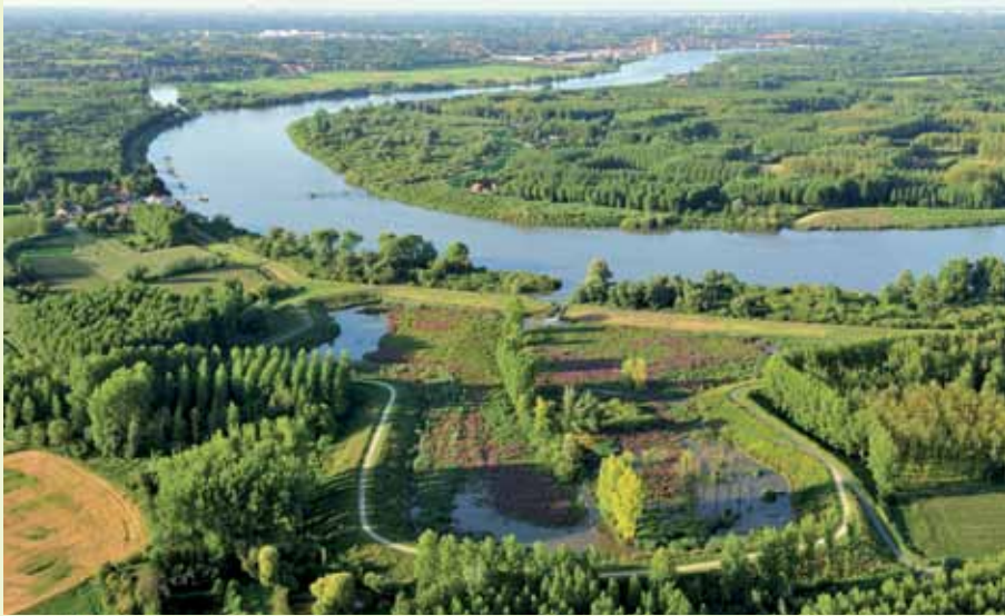
Figure 4.19. Aerial photo of the Lippenbroek
