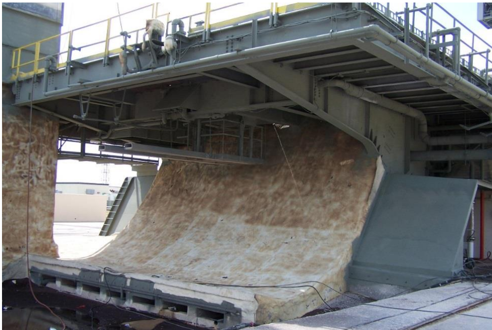
Figure 13. USAF CCAFS flame deflection trench at space launch Complex-6.
