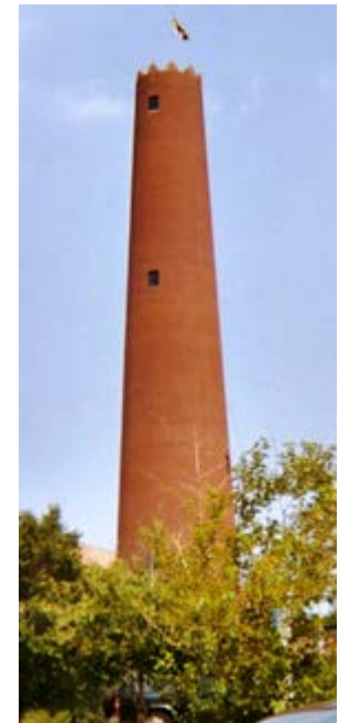
Phoenix Shot Tower Baltimore, MD, 1828 234' - tallest structure in US 2.5 million pounds shot/year
