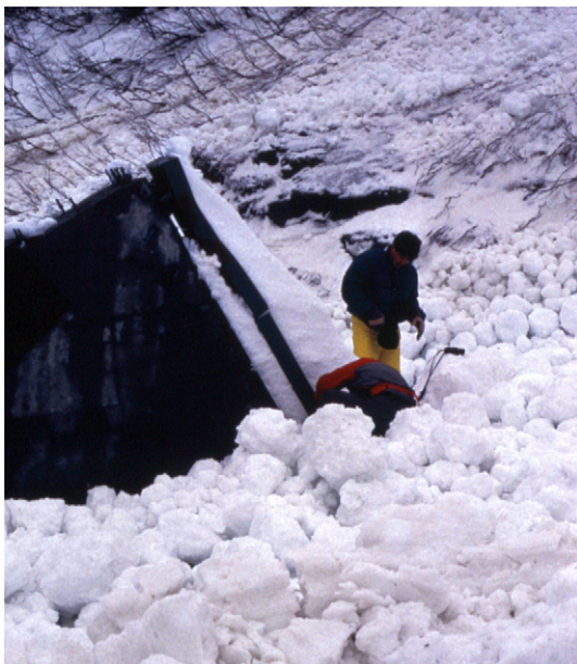
Fig. 19. Load plates LC1 (top) and LC2 mounted on the concrete wedge after a wet-snow avalanche event. LC3 is covered by deposition (Avalanche event 1991-03-20).
