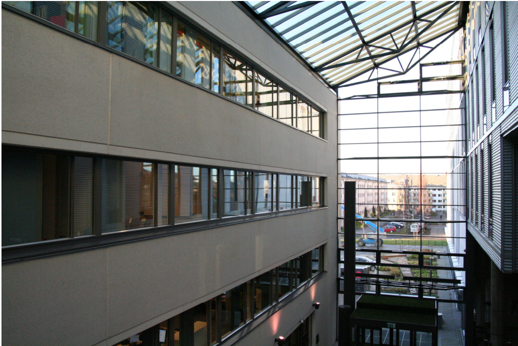
Figure 8: East façade of area measured by meter 33 (2 nd floor).
