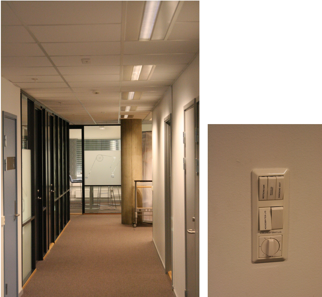
Figure 17: Interior view of the corridor space (left picture). Outside working hours the corridor lighting may be operated by a manual switch with a timer (right picture).
