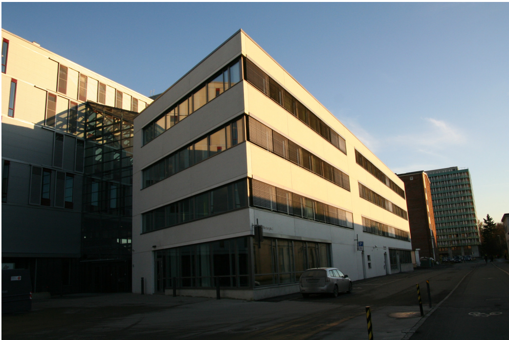
Figure 9: North and west façade of area measured by meter 33 (2 nd floor).
