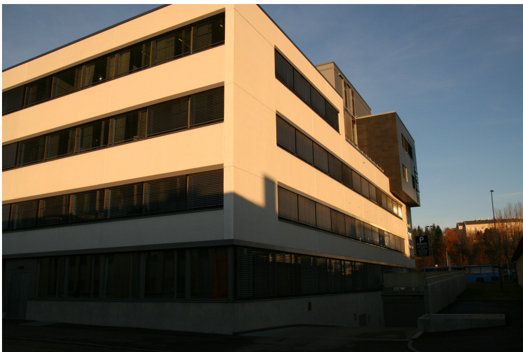
Figure 10: West and south façade of area measured by meter 35 (2 nd floor).
