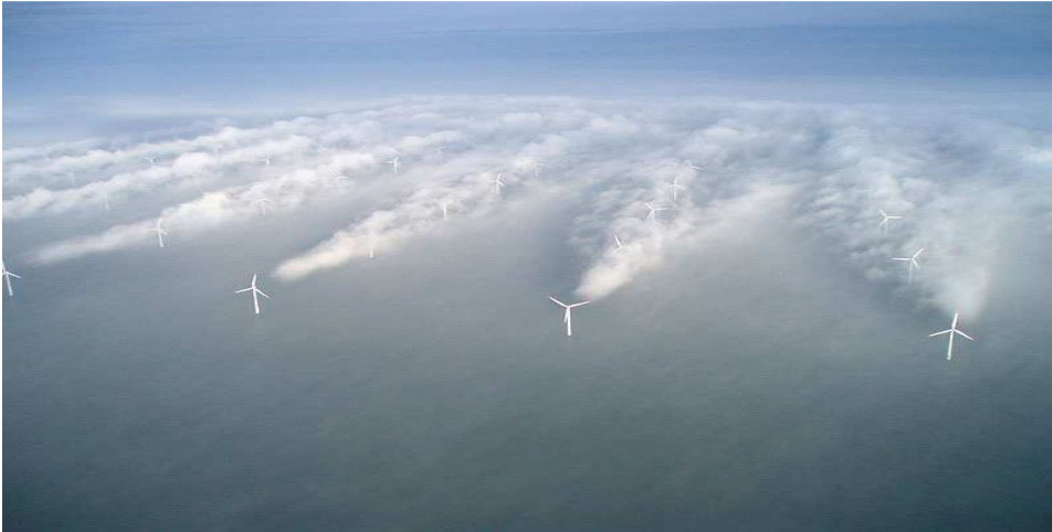
Fig 2. Natural visualisation of Wake turbulence behind wind turbines – (photo of Horns Rev offshore wind farm in Denmark) [8]
