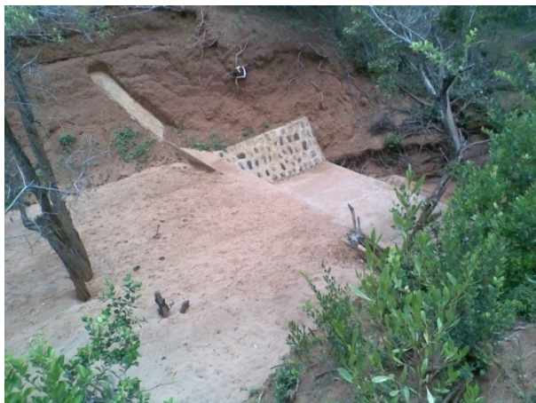
Figure 3.11 Sand dam filled with sand on upstream side (left) and water abstraction well by the side of the dam (right).
