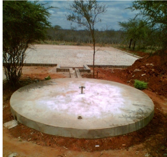
Figure.3.8 Rain water harvesting cisterns with open ground catchment provided with silt traps (left) and with paved ground catchment (right).
