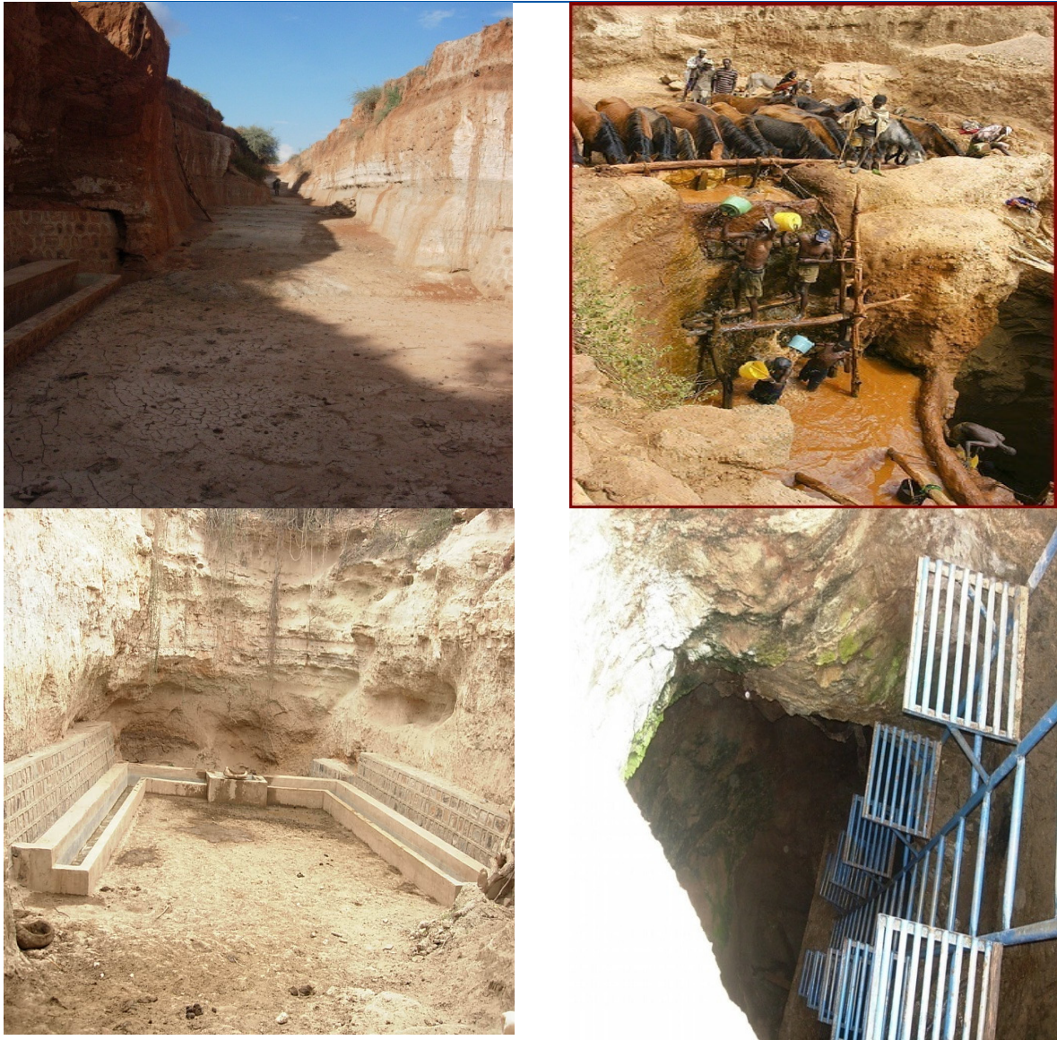
Figure 3.3 Singing wells in Borana; Entrance road (top left), People lifting water standing on wooden steps and watering livestock with mud troughs (top right), Improved watering troughs and metallic ladder and steps (bottom left and right).
