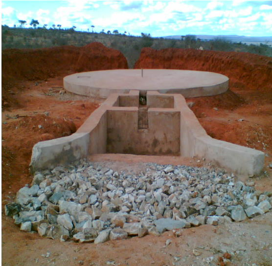
Figure.3.8 Rain water harvesting cisterns with open ground catchment provided with silt traps (left) and with paved ground catchment (right).
