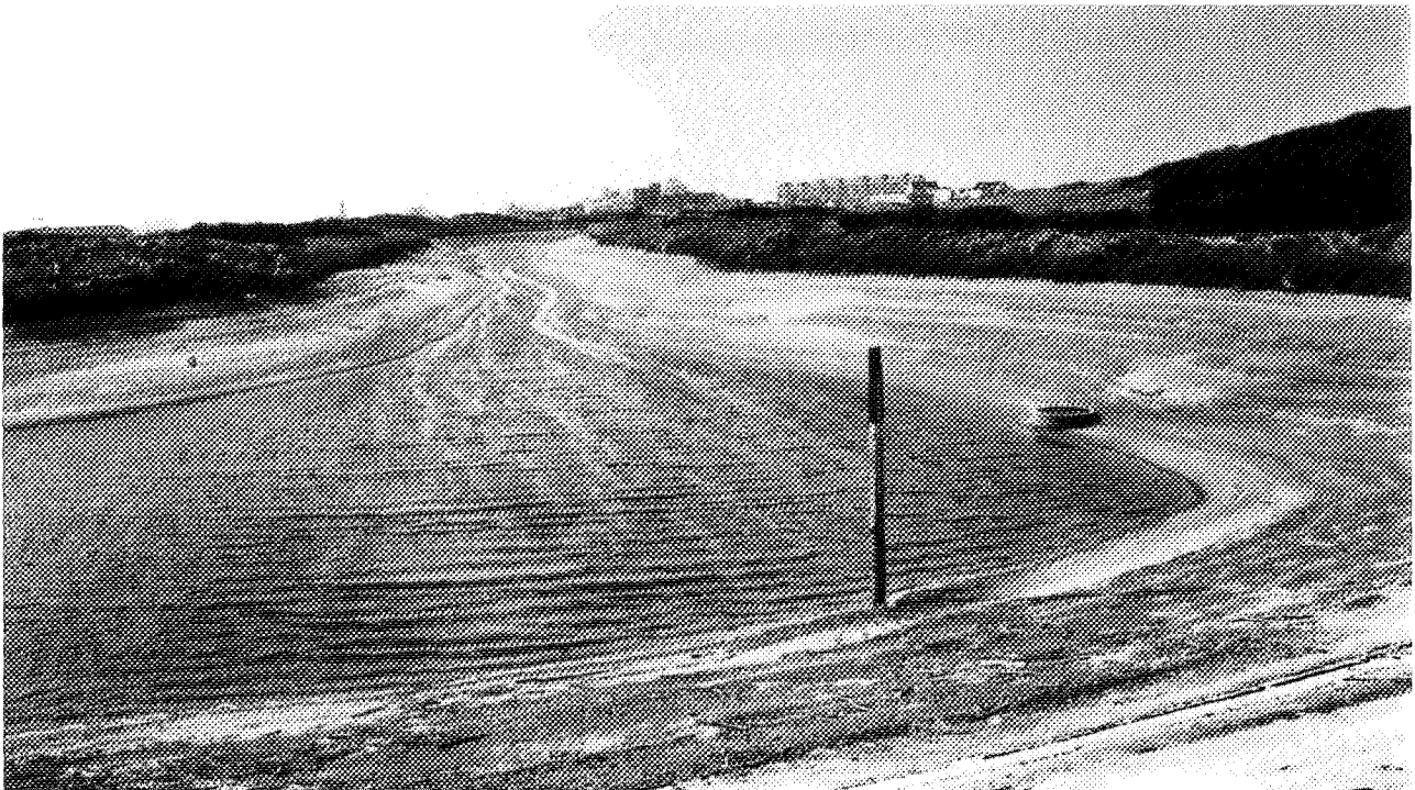
FIG. 1.5 Spreading basin 8.4.2 in the Scheveningen area during low water level. The inlet of pretreated river Meuse water can be seen on the right hand side, and the city of Scheveningen on the horizon (photo by E. Wanders, DZH-archive).
