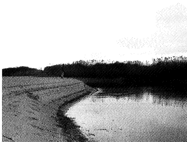
FIG. 4.12 The basin banks of a recharge basin in the Zandvoort aan Zee spreading area exposed during low water level. The intake of river Rhine water was suspended in order to exclude a pollution wave on the river. The high permeability of the sandy basin banks and low permeability of bottom sludge (Fig.4.13), may result in about 80% of all recharge passing through these banks.
