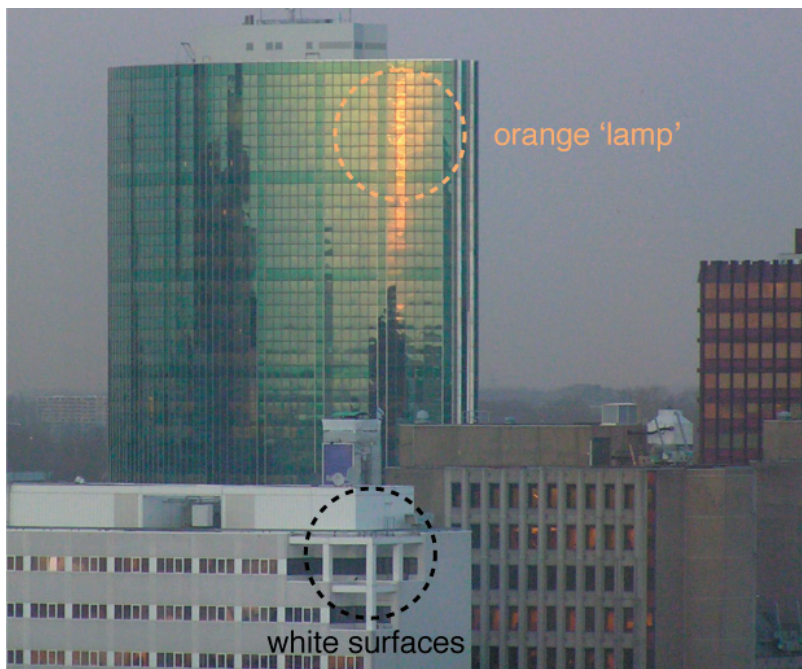
Figure 8: Would you have thought that the sun is so orange (mirror reflection in tall building) if you had only seen the lower buildings? Does this influence how you see the white surfaces?
