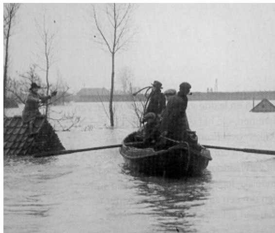
Figure 3.2 The last serious flooding of a polder along the rivers occurred in 1926 Source: Middelkoop, 1998.
