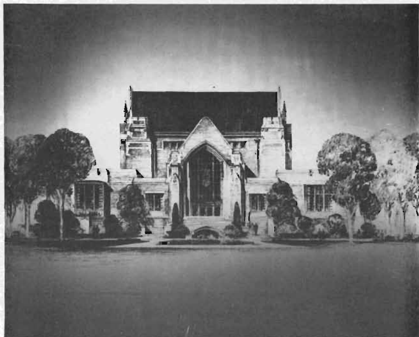
THE MARY J. BOOTH LIBRARY Under construction, 1949
