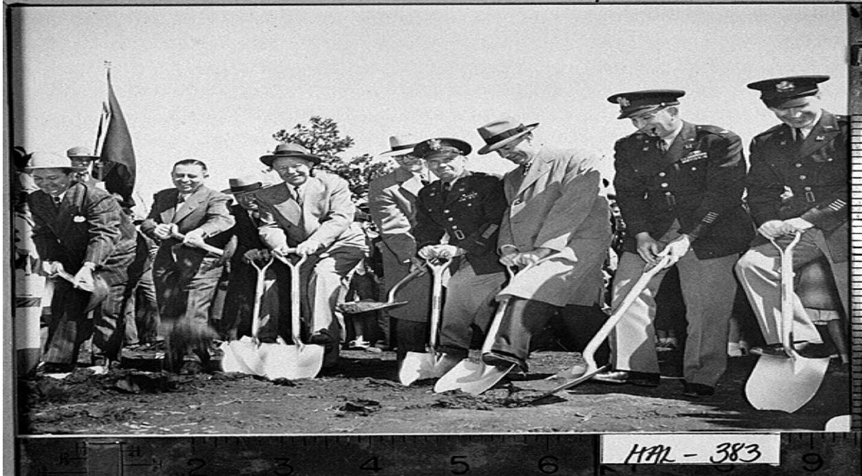
Figure 4: Photograph of Groundbreaking for Buford Dam, Georgia, 1950 Mar. 1 (to the far left is Georgia Gov. Herman Talmadge). Source: Vanishing Georgia, Georgia Division of Archives and History, Office of Secretary of State.
