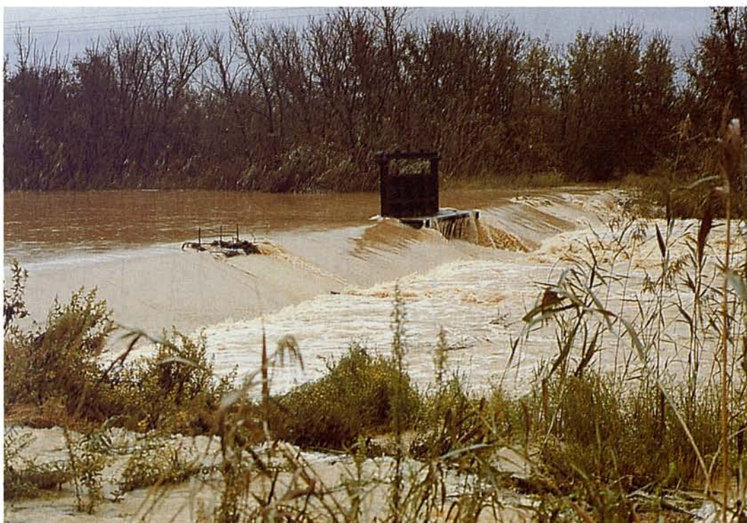
Darrer tram del Canal Gran amb la presa vessant durant una avinguda. Final portion of the Great Canal showing the dam overflowing during torrential floods. (Foto: Joan Mayol)
