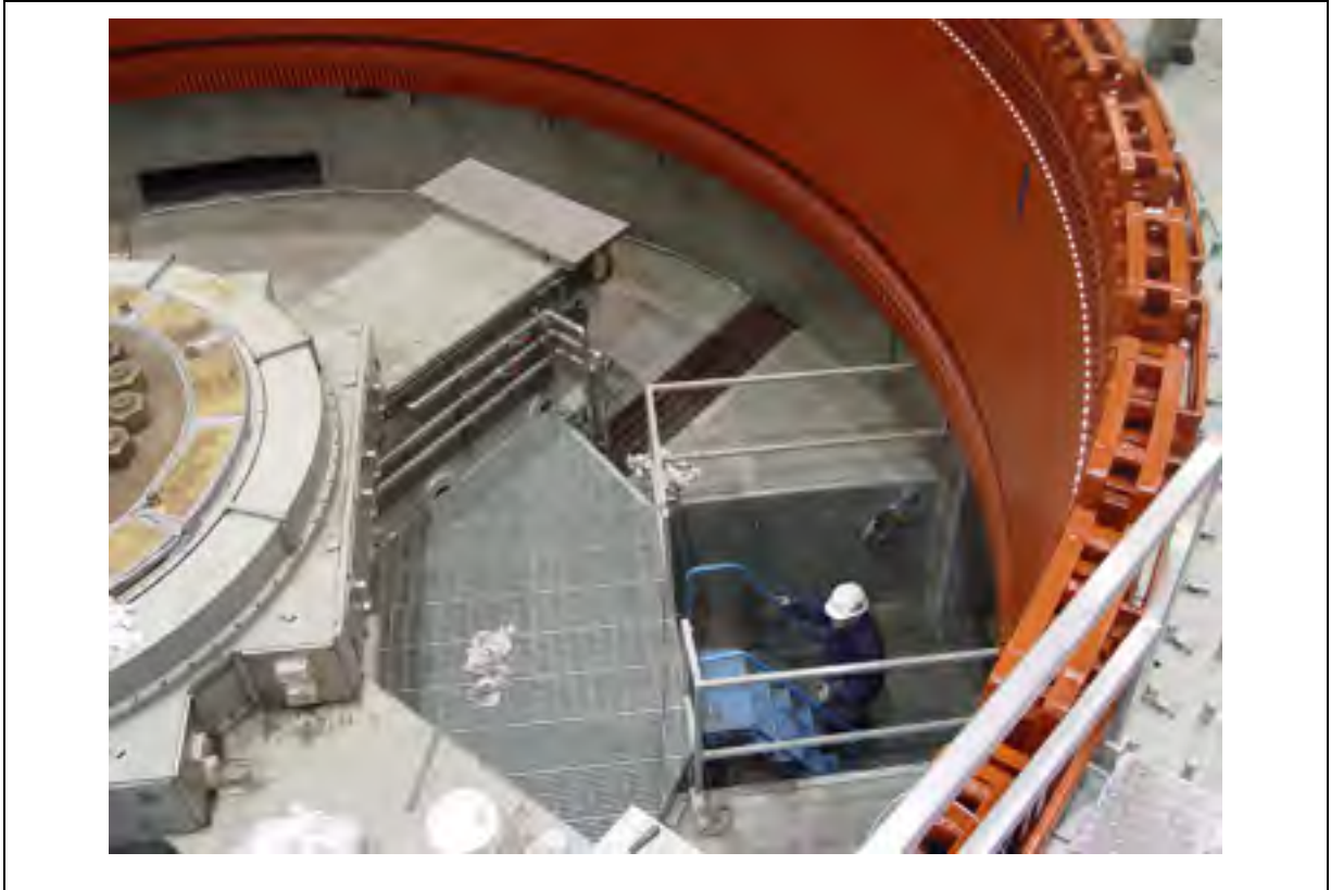
Figure 2.3 Stator of a large synchronous machine
