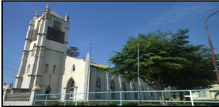
Figure 10: The first church building in Nigeria, the Cathedral of St. Peter Church in Abeokuta (Source: http://www.nairaland.com/ by Codedrock 2015)
