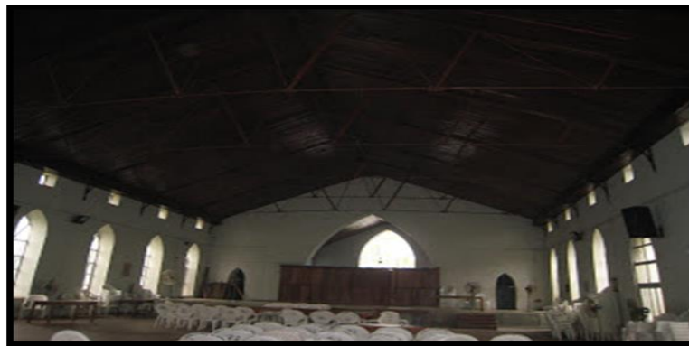
Figure 11: The interior of the first church building in Nigeria (Source: http://newhomeinlagos.blogspot.com.ng by Bod and Lisa 2009)
