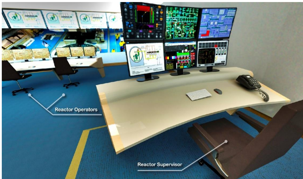
Figure 2: The main control room
