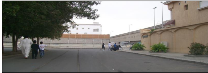
Father and his two children walking on street edge, no pedestrian path, no calming traffic elements and poor landscape
