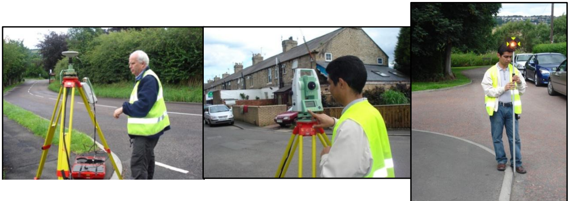
Figure 4.4 Field work using GPS to establish control points, and total station to survey the location of points
