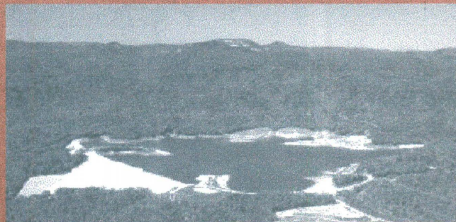
Bad Creek Hydroelectric Station
