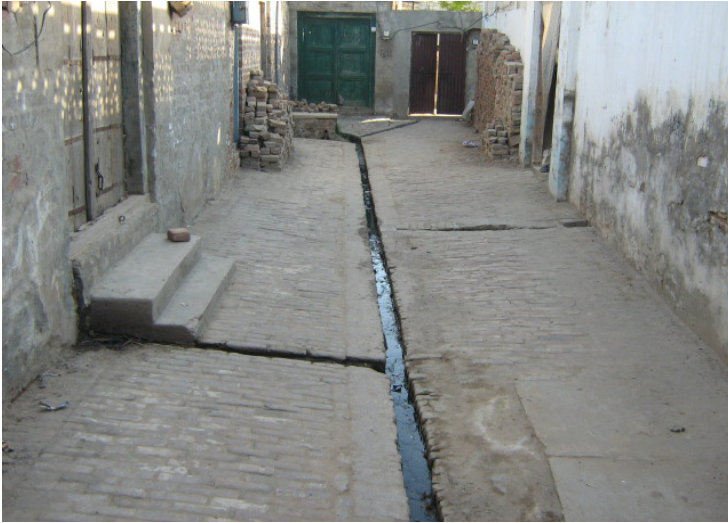
Picture 5: “naali” drainage system.
