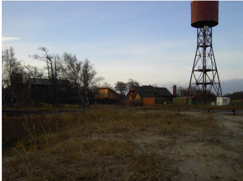
Fig. 8: New houses on the edge of the protective dune in Lesnoye(Albrecht 2007)
