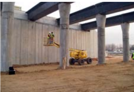
Composite bridge beams being installed on site (Madrid)
