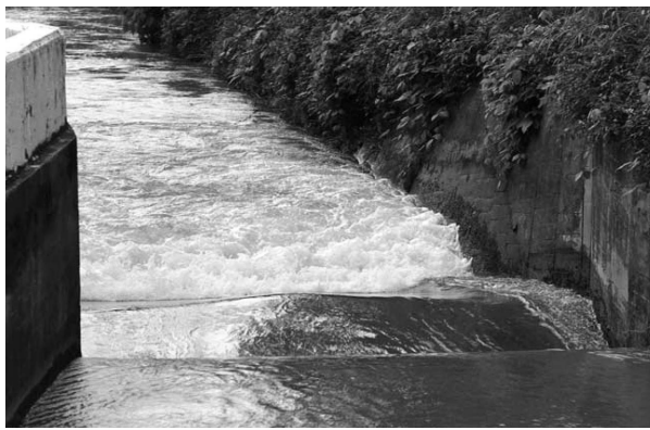
Figure 2 : Hydraulic jump in an irrigation channel at Taroko (Taiwan) on 10 Nov. 2010 – Flow from foreground right to background left
