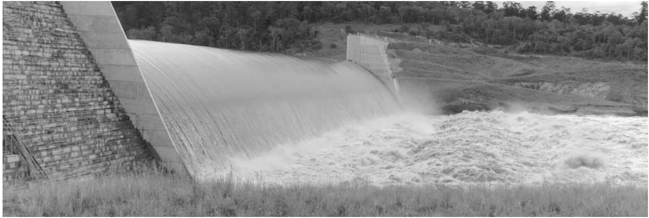
Figure 1 : Hydraulic jump stilling basin in operation downstream of Paradise dam spillway (Australia) on 30 Dec. 2010 – Q = 6,300 \text{ m}^3/\text{s} , Re = 1.9 \times 10^7
