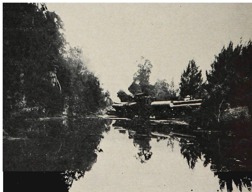
3. Low-level bridge across the Coomera River. Looking east, 5 miles from Canungra.
