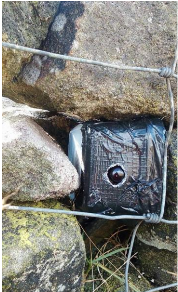
Figure 3.5c Top path sensor (In dry stone wall).
