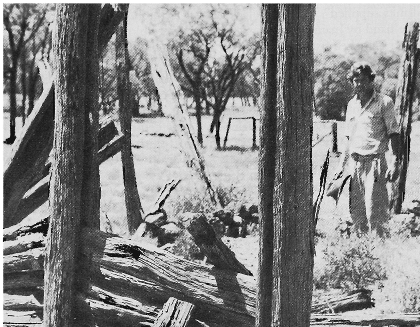
Richard Yeates, great-grandson of Sidney Yeates, stands beside fire-place ruins at old hut on Boondoon. Note the deep slots in the gidyea posts, into which the tapered ends of the horizontally laid slabs fitted.
