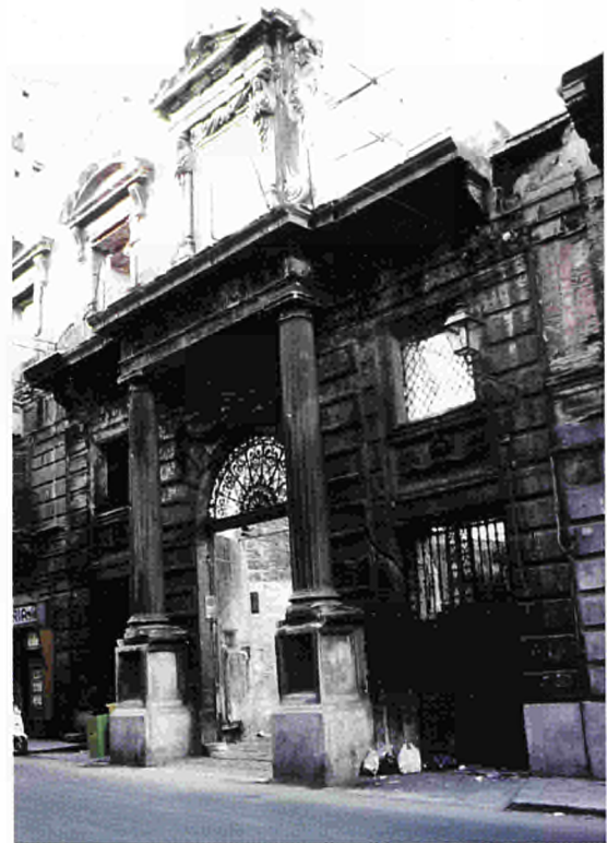
Figure 5.2: The front wall of Palazzo Geraci in Palermo (Sicily, Italy) which was remodelled in the ELSA laboratory (see Figure 5.3)
