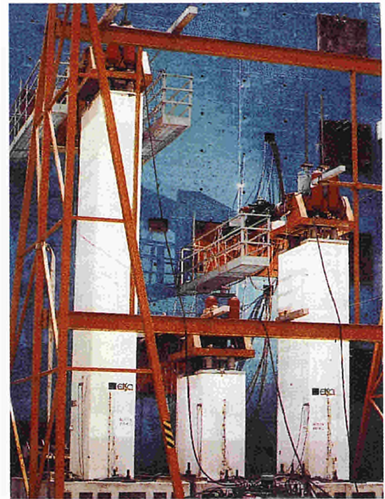
Figure 6.1: Isolated bridge columns tested at ELSA. The pseudodynamic earthquake simulation test was possible due to the substructuring technique, where the bridge-deck behaviour is simulated by the computer. The digital controllers developed at the JRC proved essential in this application.
