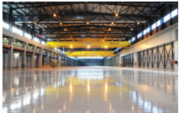
Internal view of the PF Coils building
