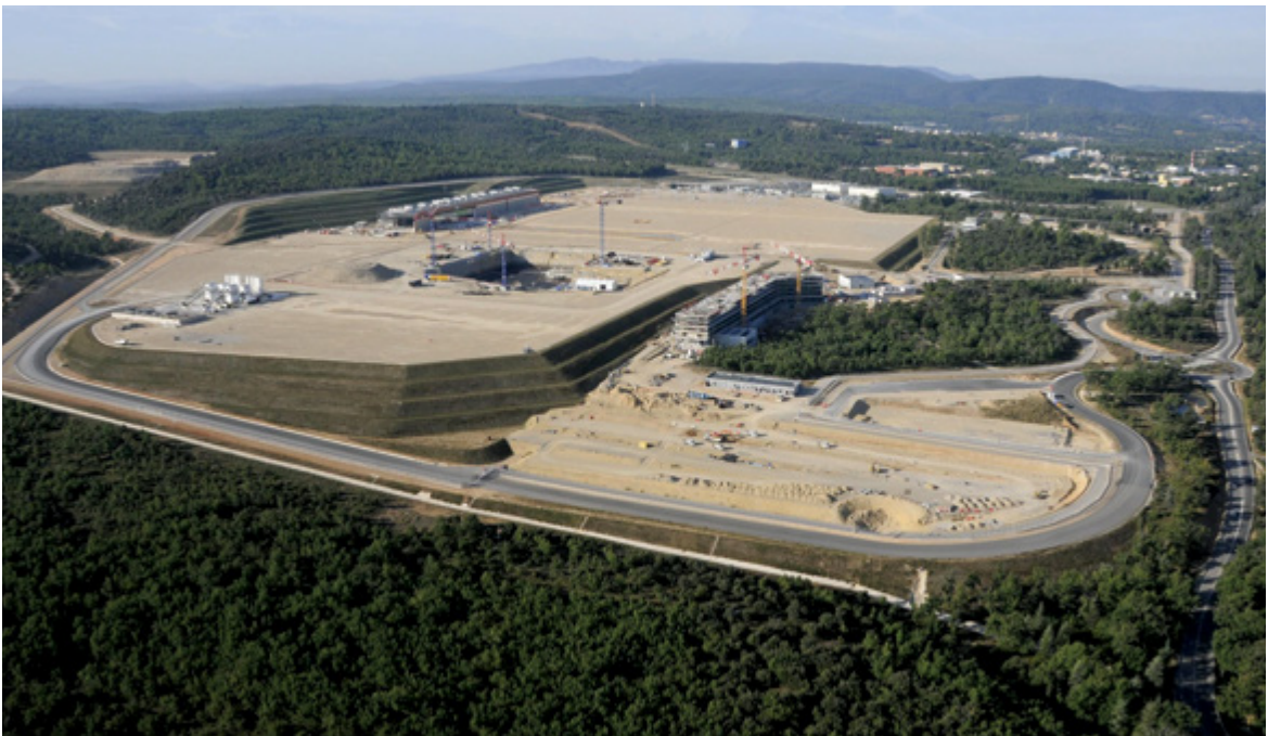
ITER platform, September 2011 (courtesy of the ITER IO)
