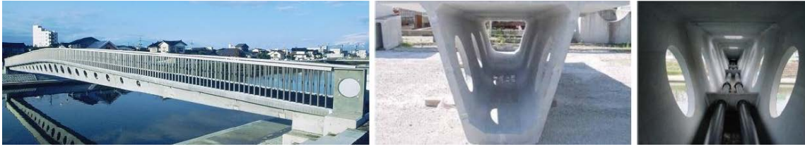
Figure 3-4: Sakata Mirai footbridge (Uchida, et al., 2014).
