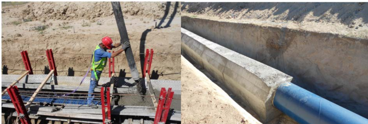
Figure 12-6: Concrete pumping and result.
