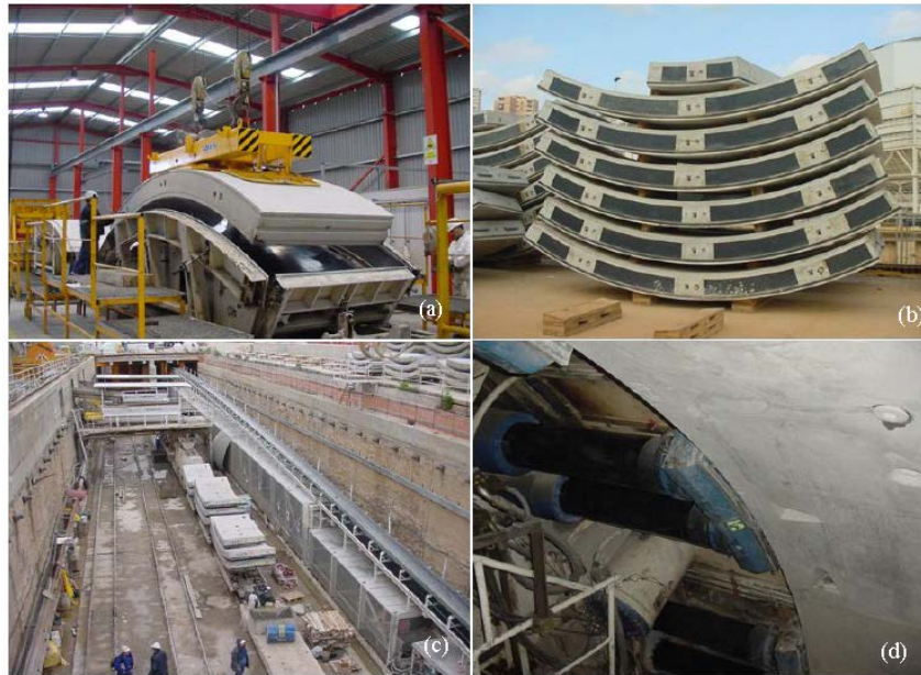
Figure 3-3: Temporary load stages of a segment (De la Fuente, et al., 2014): (a) demoulding; (b) stocking; (c) transportation; (d) thrust of the jacks.
