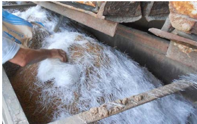
Figure 12-5: Manual fibre addition.
