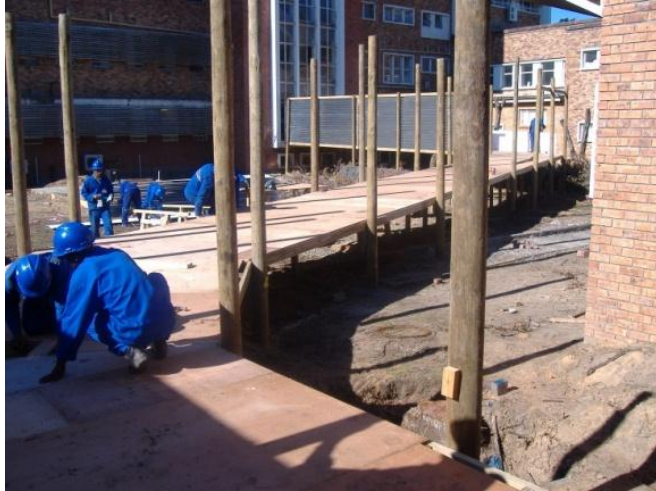
Temporary walkway under construction
