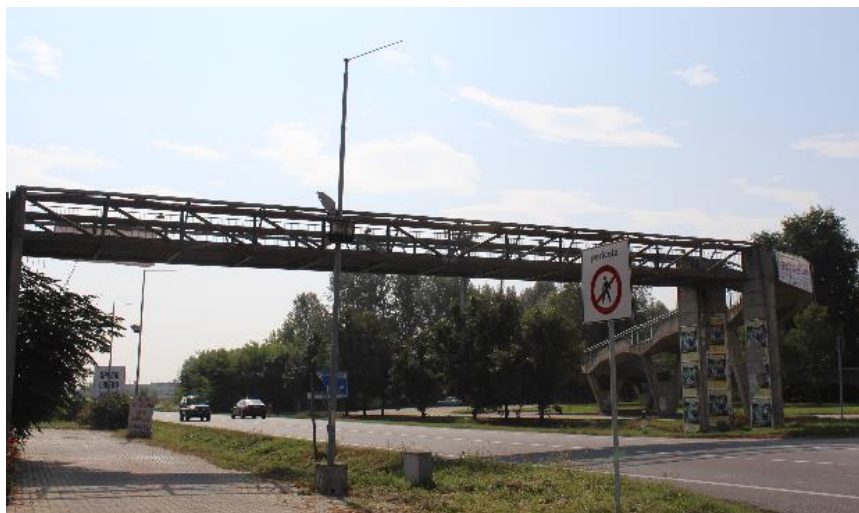
Figure 1. View to the footbridge and the road system in Villastellone
