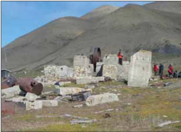
3.13 Sea-facing front of the former engine house (9). (Photo: I. West, LASHIPA 1, 2004.)
