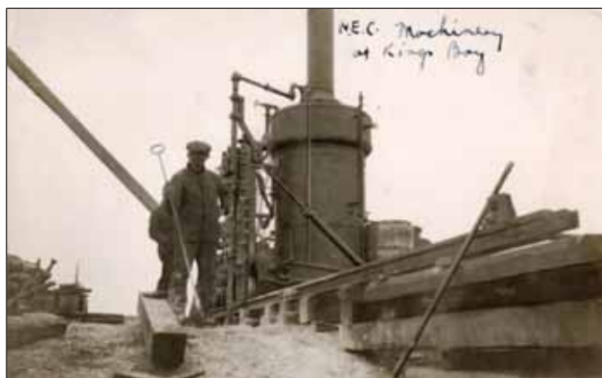
7.12 Channeler producing a cut at No. 3 Quarry in 1912. (Source: pol02979, Polar Museum, Tromsø.)
