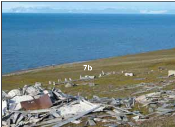
3.12 The foundation of the lowest lying building in the settlement (7b) was made of timber piles. (Photo: I. West, LASHIPA 1, 2004.)
