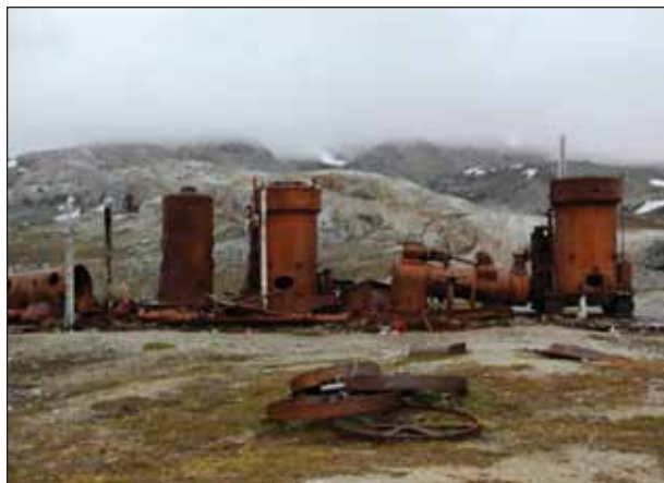
4.47 Machinery and equipment to extract marble in the former workshop (4) on Marble Island. (Photo: D. Avango, LASHIPA 5, 2008.)
