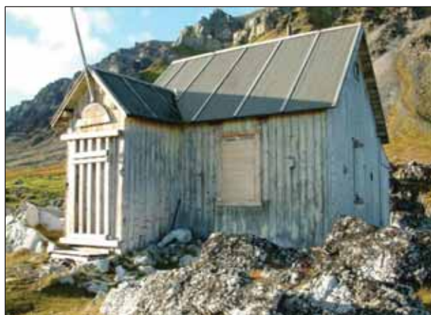
4.16 Pre-fabricated staff house at Camp Millar. (Photo: U. Gustafsson, LASHIPA 3, 2006.)
