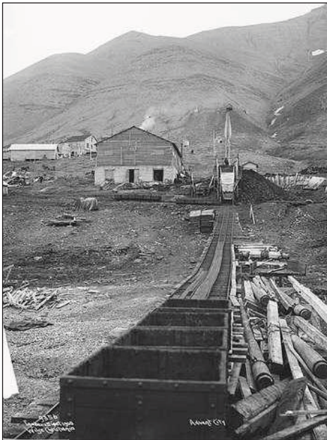
5.17 The self-acting incline, the coal tip, and the engine house. Note the smoke coming from the plant. (Source: Wilse, A. B. (1908) NF.W 09356. Galleri NOR [Online]. Available at: http://www.nb.no/gallerinor/index.php (Accessed: 21 September 2011).
