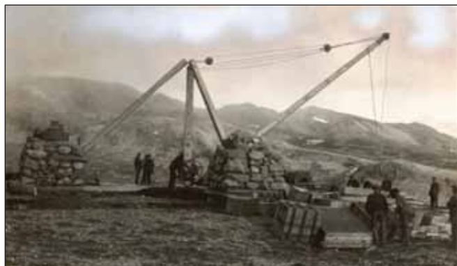
7.6 One of the two cranes made by John M. Henderson & Co. of Aberdeen, which were delivered to Marble Island in 1911. (Source: pol02970, Polar Museum, Tromsø.)
