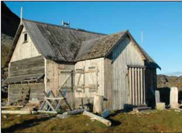
4.17 Pre-fabricated worker's barrack at Camp Millar. (Photo: D. Avango, LASHIPA 3, 2006.)
