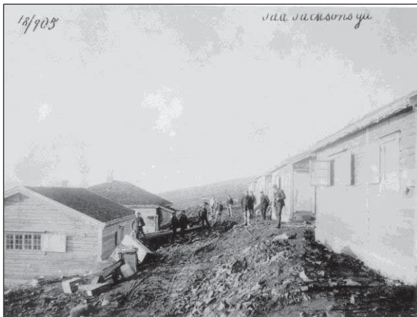
5.13 Four barracks, Huset, and the store in 'Ida Jackson Street' in mid-September 1905. Due to limited space, the ground had to be levelled first. Note the cart tracks in the street. (Source: Photo Library np002339, Norwegian Polar Institute, Tromsø.)
