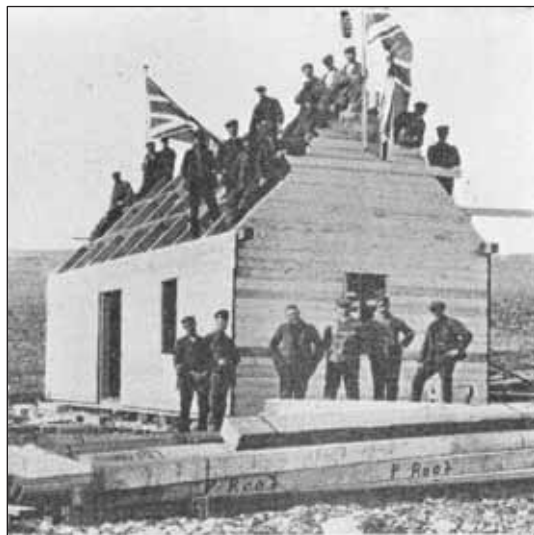
7.3 Workers flying the Union Jack at both ends of a pre-fabricated barrack on Marble Island in 1911. (Source: Marble Island (1913). 443-A, British Geological Survey, Keyworth.)
