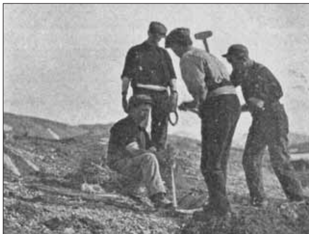
7.7 Drilling to place a shot into marble. (Source: Marble Island (1913) 443-A, British Geological Survey, Keyworth.)
