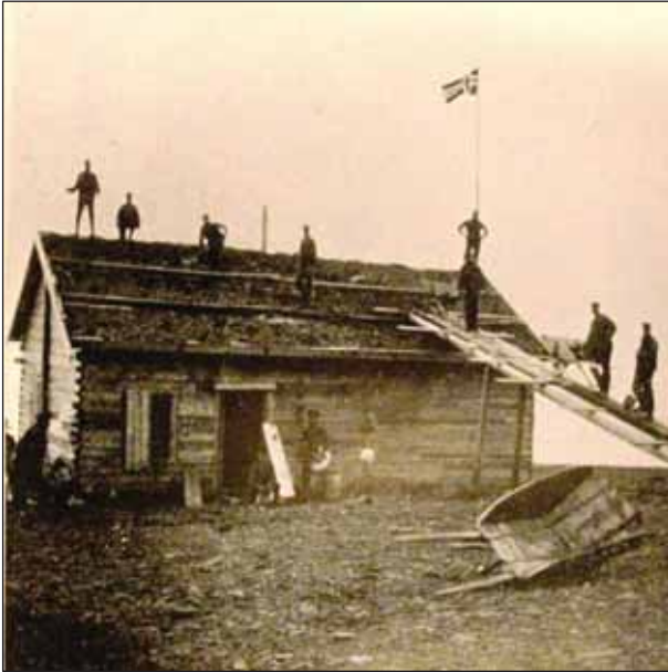
6.15 Michelsenhuset under repair in 1906. Note the independent Norwegian flag. (Source: The Northern Exploration Company, Ltd. (1911) The Northern Exploration Company, Norwegian Polar Institute, Tromsø, p. 122. )
