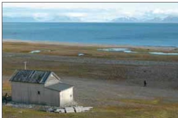
3.35 The reconstruction of Camp Bell. Note its former location at the shore on the far right. (Photo: D. Avango, LASHIPA 3, 2006.)
