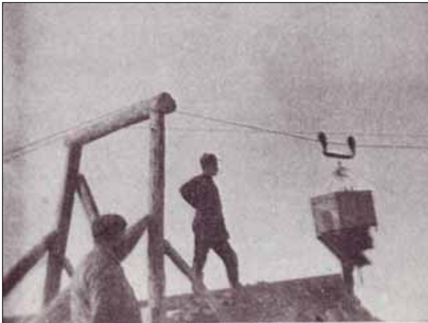
5.4 Lower terminus of the ropeway, coal dumping being in progress. (Source: Hoel (1967a) p. 557.)
