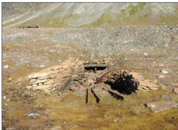
4.19 Collapsed mine entrance at Camp Miller. Note the mine tubs in the top left corner. (Photo: U. Gustafsson, LASHIPA 3, 2006.)
