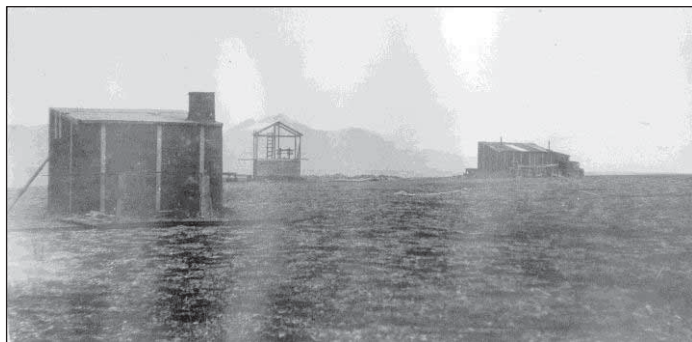
7.30 Shaft as well as workshop and house at the Icefiord Lead and Zinc Mine. (Source: Photo Library np001973, Norwegian Polar Institute, Tromsø.)
