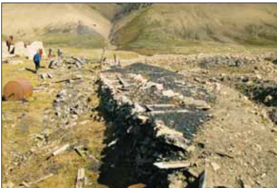
3.9 Short railway embankment (3b) with wooden sleepers and a thin spread of coal. (Photo: M. Oglethorpe, LASHIPA 1, 2004.)
