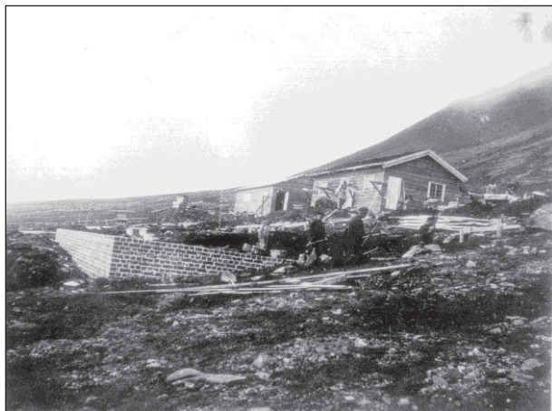
5.11 Two pre-fabricated workers' barracks and the brick foundation of Huset in 1905. (Source: Photo Library np002341, Norwegian Polar Institute, Tromsø.)
