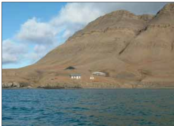
3.20 Overview of Camp Morton. Obvious anthropogenic features included two houses and a stockpile of coal. Note the traces of coal up the mountain. (Photo: U. Gustafsson, LASHIPA 3, 2006.)
