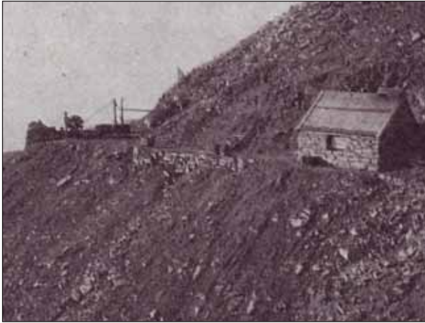
5.3 Levelled space at pithead creating room for railway tracks, winding gear, and a stone-built smithy. (Source: Hoel (1967a) p. 560.)
