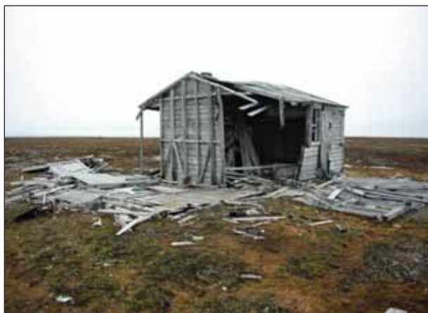
4.68 The southern section of the pre-fabricated Kenmore hut had collapsed, while northern one remained upstanding. (Photo: D. Avango, LASHIPA 5, 2008.)
