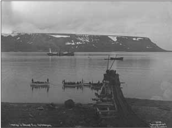
5.16 A small pier at the edge of the water. Note the parallel tracks of the self-acting incline. (Source: Wilse, A. B. (1908) NF.W 09358. Galleri NOR [Online]. Available at: http://www.nb.no/gallerinor/index.php (Accessed: 21 September 2011).
