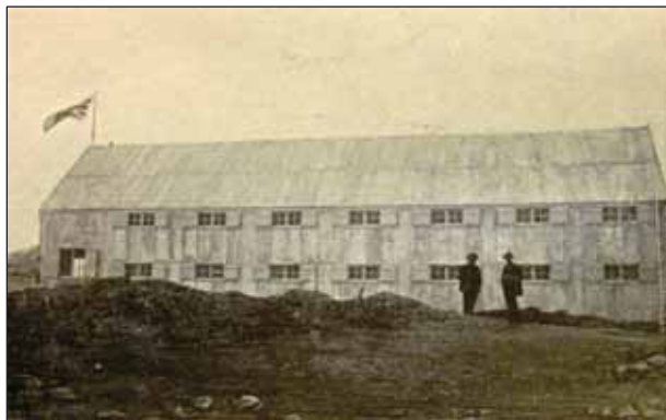
7.13 The storehouse built in 1913 was made of galvanized iron. Note the Union Jack. (Source: Some particulars (1914) Northern Exploration Company (N.E.C.), Norwegian Polar Institute, Tromsø.)
